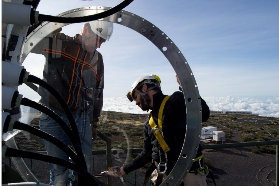
Figure 15: Removing Front Lid.
