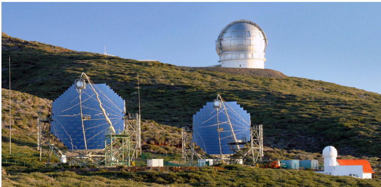
Figure 3.1: Picture of the MAGIC telescopes on the Roque de los Muchachos observatory. From left to right we have MAGIC-I, MAGIC-II and the counting house (the data taking building) with the LIDAR dome on top. The large structure seen in the background is the Gran Telescopio de Canarias (GTC). Image credit: Robert Wagner.
