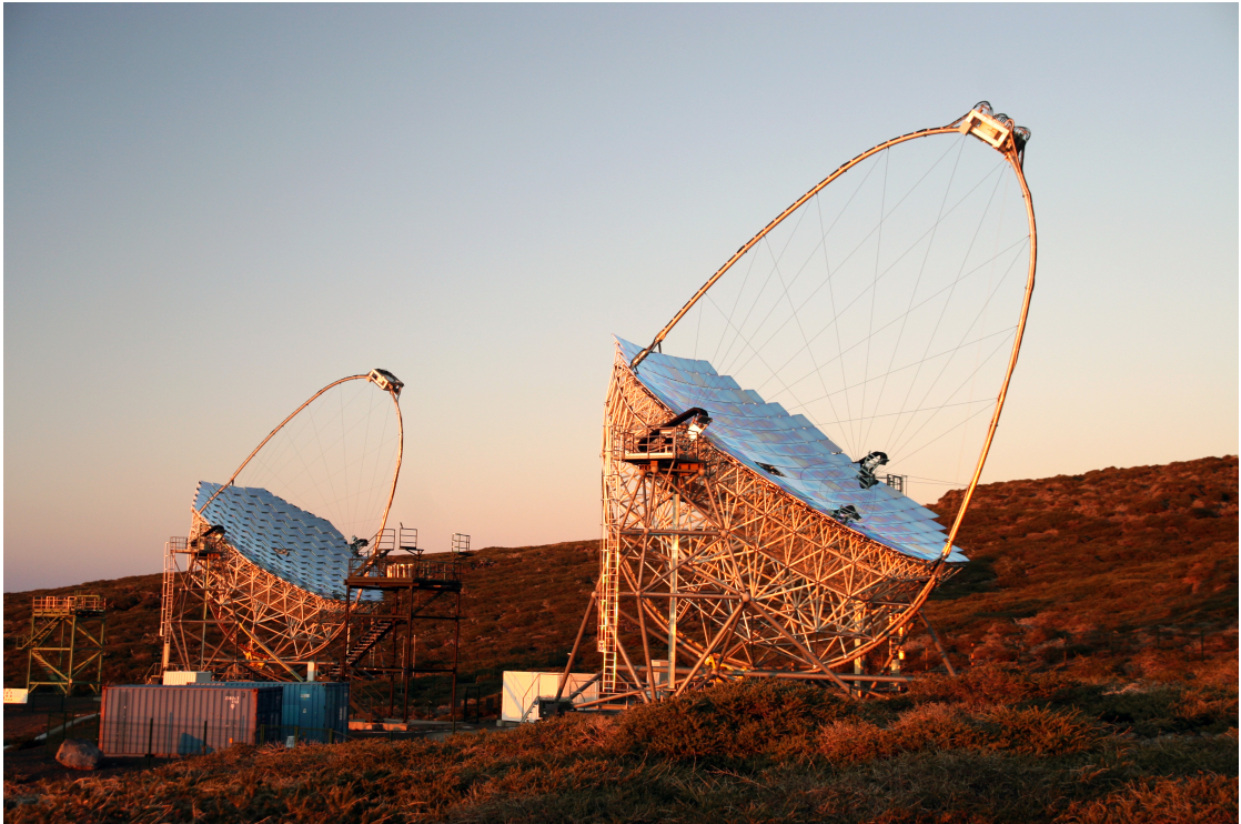
Figure 2.7: The two Major Atmospheric Gamma-Ray Imaging Cherenkov (MAGIC) telescopes, on site at around \sim 2200 m altitude on the Canary Island of La Palma. They represent one of the three worldwide currently operative IACT arrays. Each telescope features a reflector dish of 17 m diameter, supported by a light-weight structure and connected to a PMT -based camera via an arc. Photo from https://magic.mpp.mpg.de/gallery/pictures/tn/IMG_2520.JPG.html .
