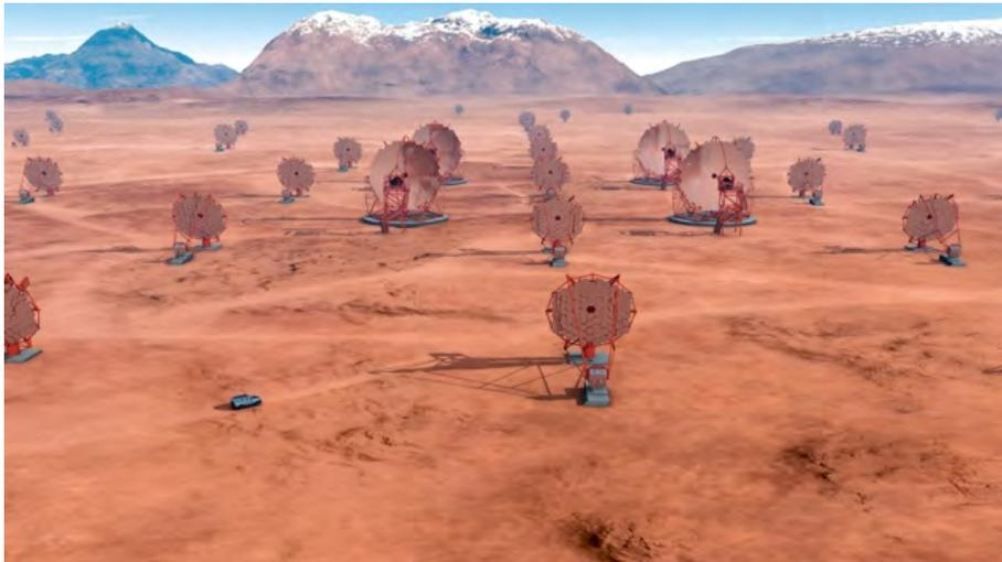
**Figure 1.7.:** Design study of the Cherenkov Telescope Array. The core of the array will consist of four large size telescopes with a low energy threshold. They are supplemented by a large number of mid and small size telescopes to cover a large area and to increase the sensitivity (design study from [13]).
